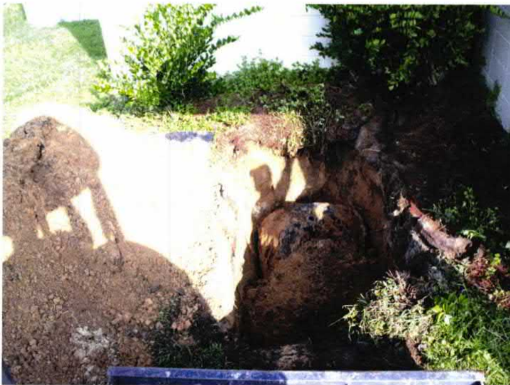
Picture 2: UST 722Bluebell excavation in progress.
